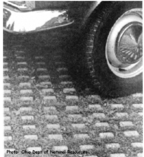
Photo: Ohio Dept of Natural Resources Concrete grid pavement
