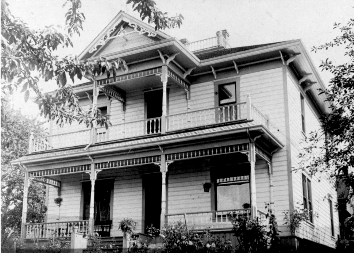
Figure 22 Example of a hip roof porch on the Henry Kraus house located at 21544 Liberty Street. Highly stylized hip roof porches were typical on Post-Colony Victorian houses.
