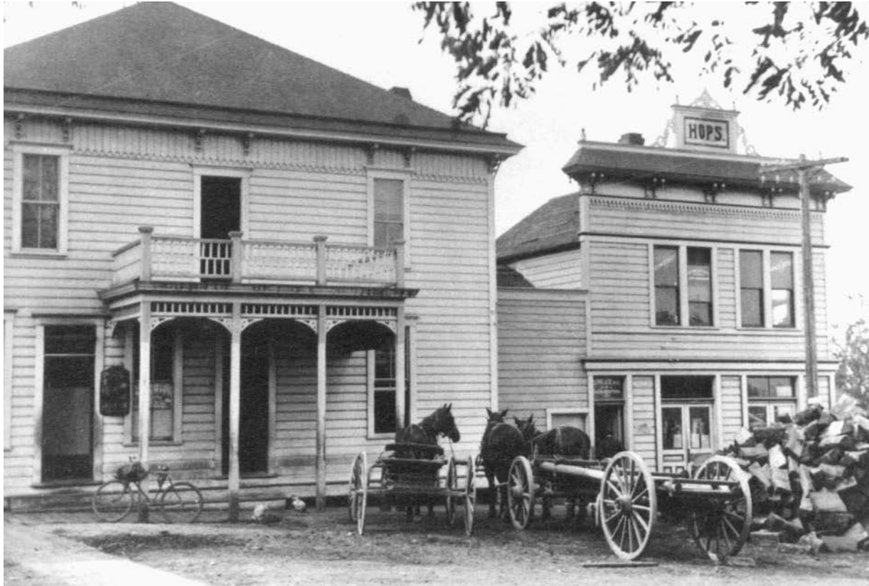
Figure 24 Located on the northwest end of Main Street, the building on the left was the “New Aurora Hotel” (circa 1895). The building on the right, closer to the railroad track providing convenient shipping, was constructed to handle the new hop brokerage business that developed after the Colony period ended. Both buildings were destroyed around 1960.
