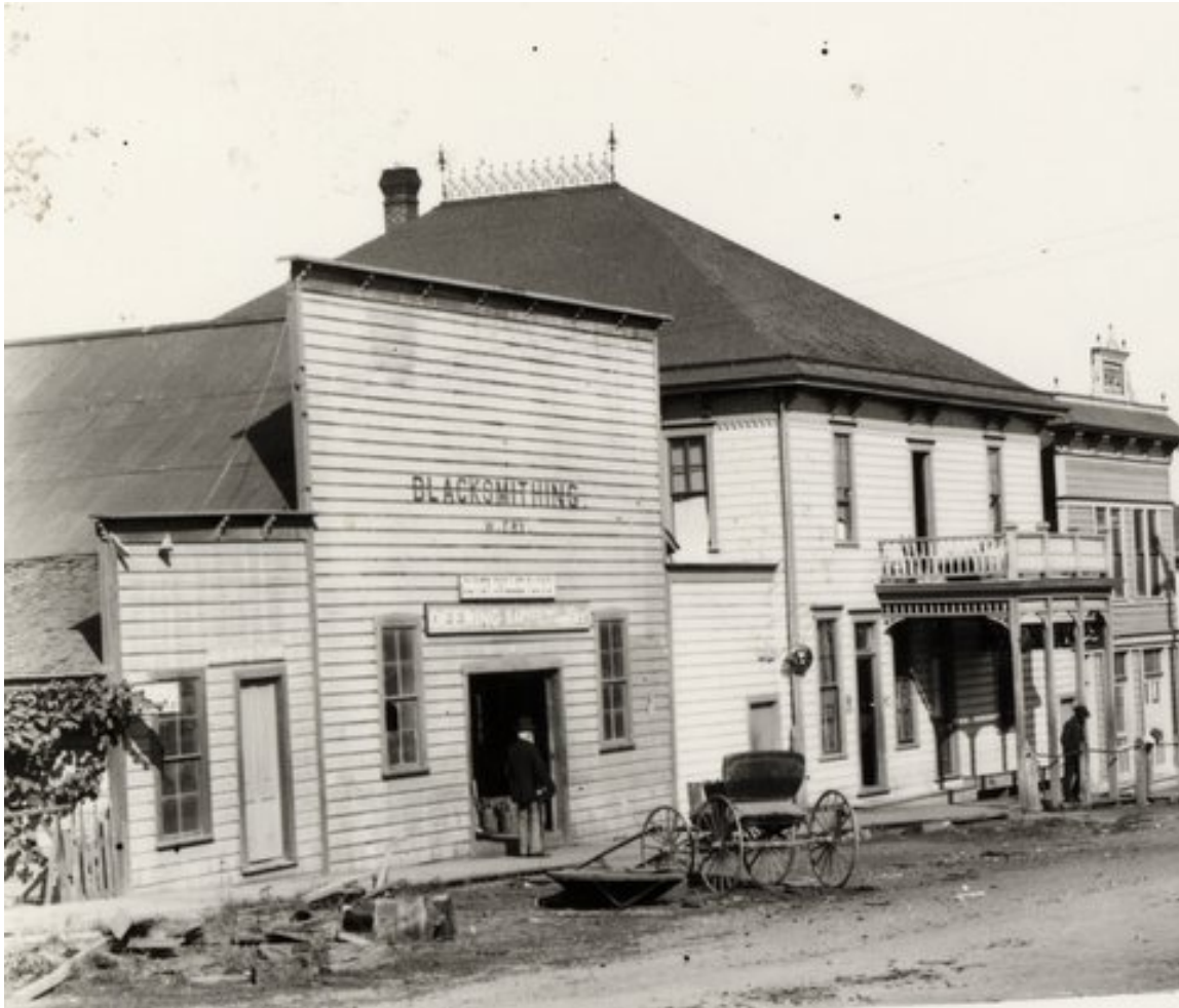
Figure 30 The Fry Blacksmith Shop, 1867 illustrates how a false front becomes a decorative parapet hiding a pitched roof in order to give the appearance of a larger commercial style building. Note that even though a workshop, there was some decorative trim. This was located next to the Walter Fry house on Main Street.
