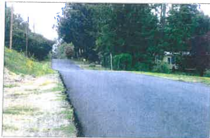
Road condition at final inspection (2016)
