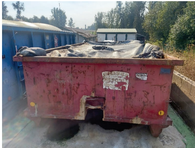
FIGURE 4-5: SLUDGE DEWATERING BAGS
