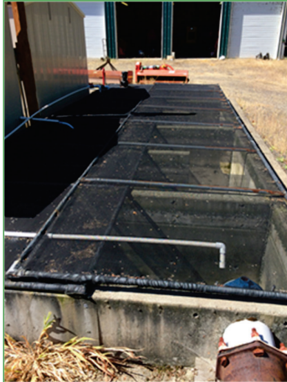
Chlorine Dosing System
