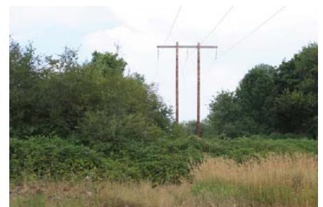
Existing overhead power lines running through the site.
